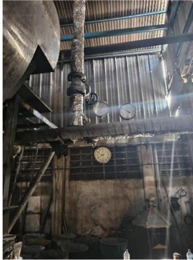
**Gambar 5 - Pipa Radiator Yang Terhubung Dari Boiler Ke Ruang Oven**
